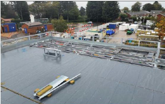
BECV: Roofing progress. Panels nearly completed
