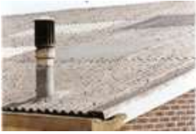
Fig 3: Asbestos cement roof panelling.
