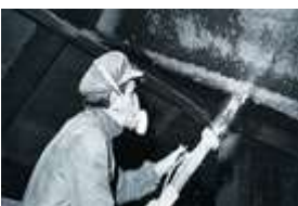
Fig 3: Under roof spray coating.
