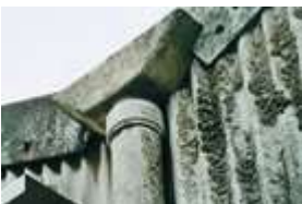
Fig 1: Asbestos cement downpipe, hopper, and profile sheet.
