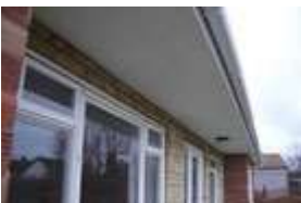
Fig 2: AIB soffit under roof
