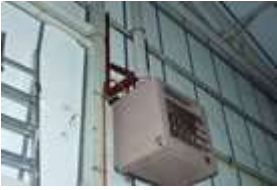
Fig 2: Asbestos cement flue from ventilation unit.
