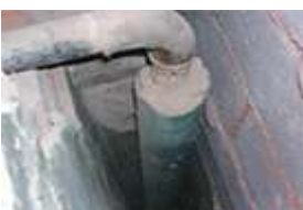
Fig 2: Lagged pipe in cavity wall.
