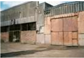
Fig 4: Asbestos cement wall panelling on warehouse.
