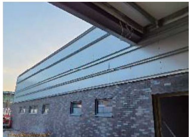
New Build – Rain Screen cladding rails being installed
