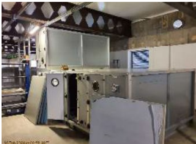
Refurb – First Floor Plant Room - ATC / CAU air handling unit delivered and being installed
