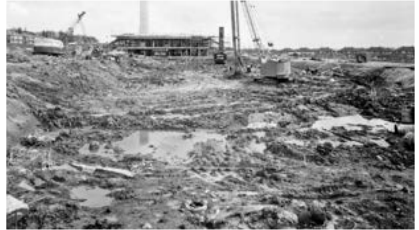
Clearing the ground for the East Ward Block, with Dining Room under construction behind, March 1964.
