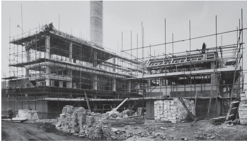
The Boiler House and chimney, January 1964.
