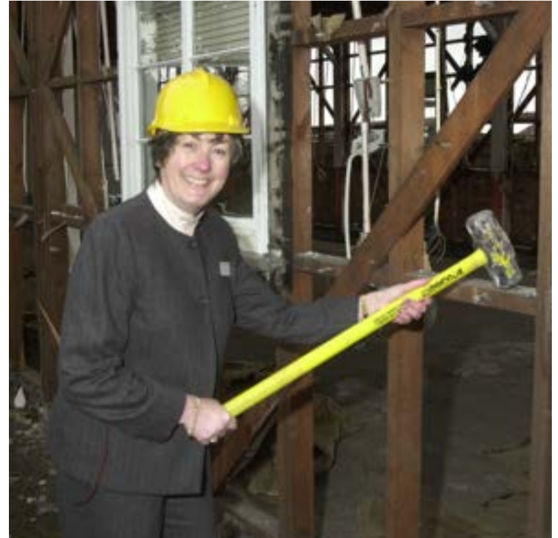
Mrs Margaret Cox, Trust Chairman, lends a hand to demolish the huts.
