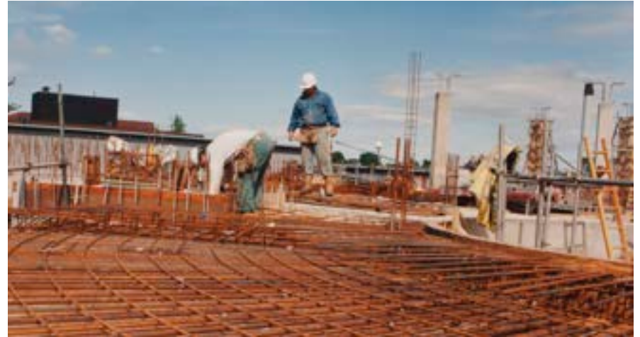
Complicated steelwork forms the roof of Montagu Hospital's new Outpatient Department.
