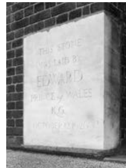
Thorne Road infirmary's foundation stone.
