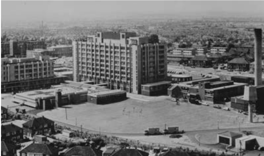
The DRI site from the south east in 1969, showing the grassed area on which the new Children's Hospital was built (see right).
