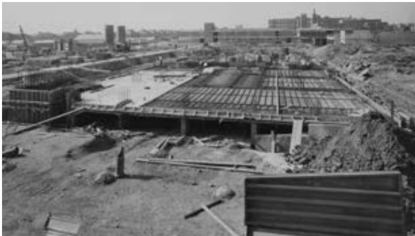
The lower floors of the East Ward Block, looking west, with the 1930 infirmary in the distance, September 1964.
