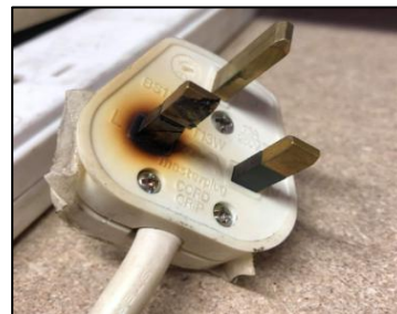
Plug top showing signs of overheating
